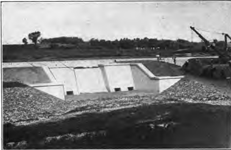
FIG. 102.—Siphon spillway, Champlain division, New York State Barge Canal.
